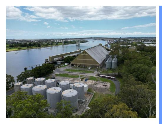
QBT is a bulk storage and handling facility with the capacity to sample, test, receive, store, pack and ship a range of grains and liquids. These include, but are not limited to wheat, sorghum, maize, pulses, tallow, edible oils, and propylene
